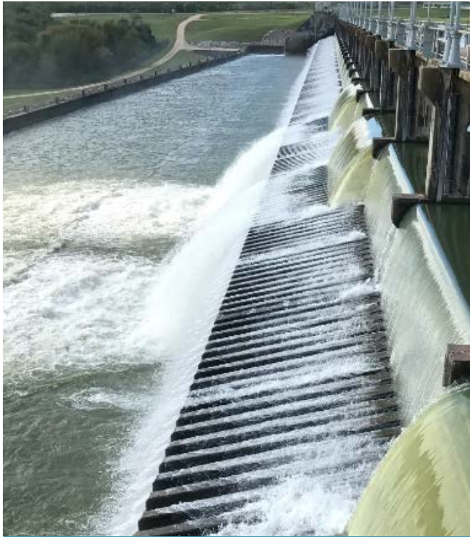
Flood gates at Lake Corpus Christi, May 2019
